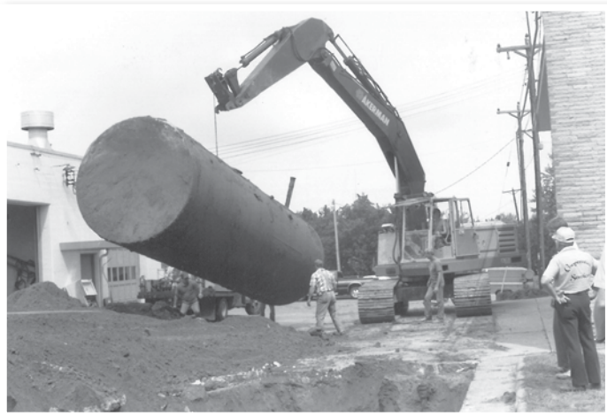
To comply with new state and federal regulations concerning underground fuel tanks, Clark Electric removed all its underground tanks. Pictured is equipment from David Laird Enterprises of Cornell, a subcontractor of McCutchin Crane Service from Dodgeville, removing a 10,000-gallon fuel oil tank. In addition to this tank, a 1,000-gallon tank, two 500-gallon tanks, and one 100-gallon tank were removed. Total cost to remove them, refill the area, and replace the concrete was more than $13,000. Clark Electric later installed a 2,500-gallon fuel oil tank inside the building for heating needs.
